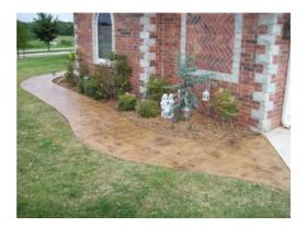
Concrete Overlay colored with 649 pigment and 680 Concrete Antiquing Stain. Sealed with AC1315 High Gloss Sealer (Photo Courtesy of Decocrete)
